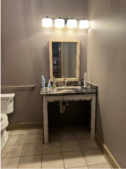
Women's Restroom Sink
