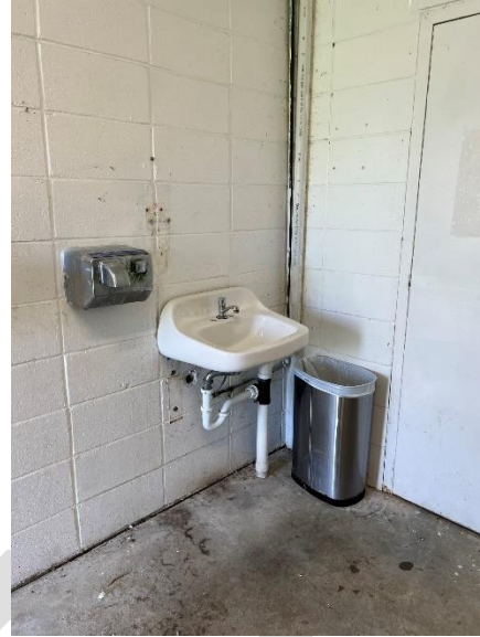
Women's Restroom Sink (2)
