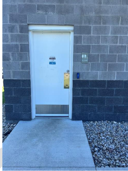
Outside Unisex Restroom Door (1)
