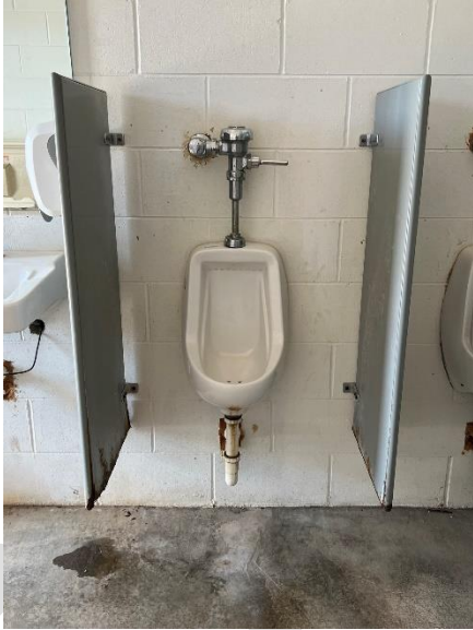
Men's Restroom Urinal (1)
