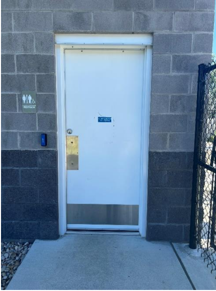
Outside Unisex Restroom Door (2)
