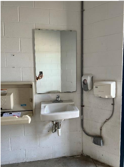
Women's Restroom Sink (1)
