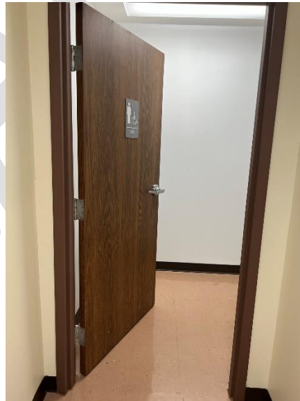
Men's Restroom Door (200 Hall)
