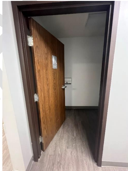
Women's Restroom Door (100 Hall)
