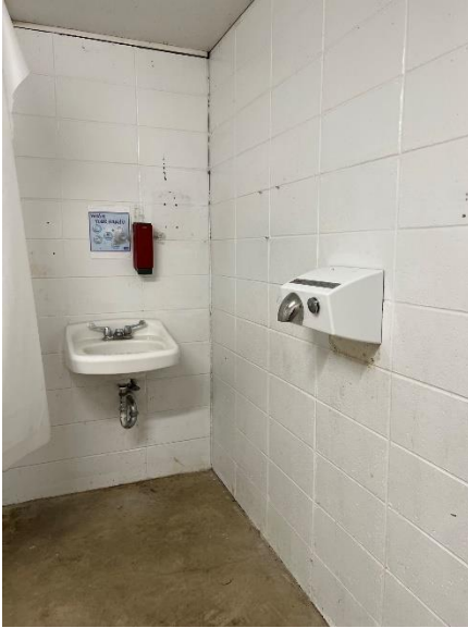
Women's Restroom Sink (3)
