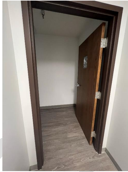
Men's Restroom Door (100 Hall)
