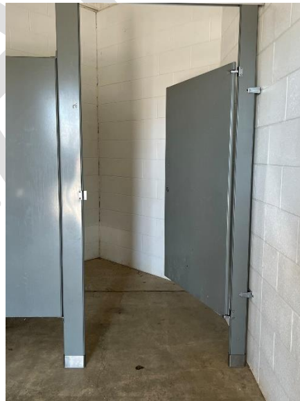
Men's Restroom Stall Door (1)
