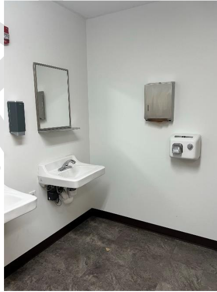
Women's Restroom Sink (Ivy Tech)
