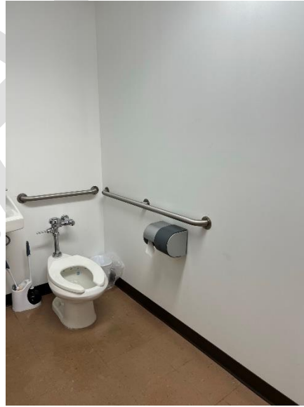
Women's Restroom Stall (200 Hall)
