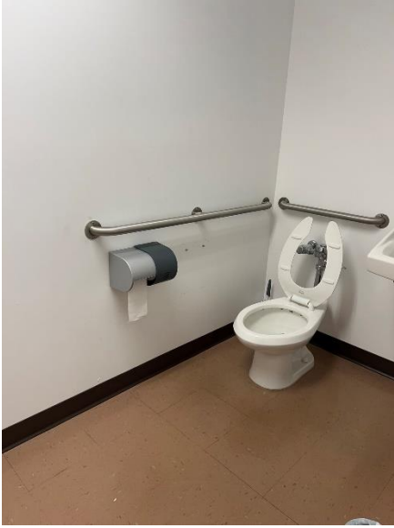
Men's Restroom Stall (200 Hall)
