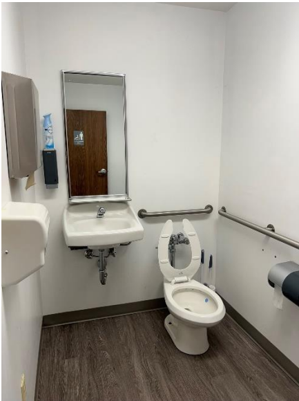
Men's Restroom Stall/Sink (100 Hall)
