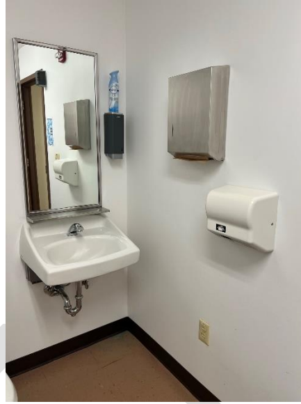
Men's Restroom Sink (200 Hall)
